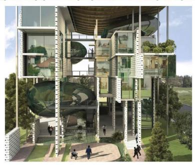
The parasol roof like an upturned basin, collects rainwater that is stored in the Underground reservoir surrounding the entire basement perimeter not only bringing the ambient temperature there but providing sufficient Drinking water to take care of the requirement of the entire office for all the year round.
